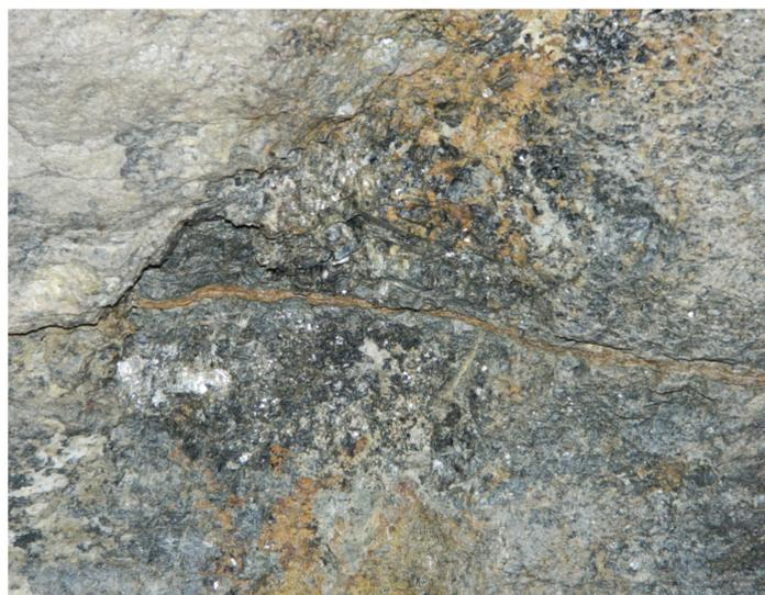
**Fig. 12.** Crystalline schist and gneiss in the shaft tunnel wall.
